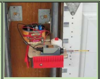
The first step was to build a platform to hold the limit switch, alarm and battery pack. A piece of ¼ inch plywood was cut to the shape required. A metal "L" bract was attached to the platform and then screwed into the wood panel between the doors.
